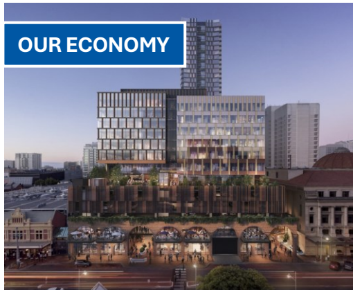
Central Market Arcade Redevelopment
