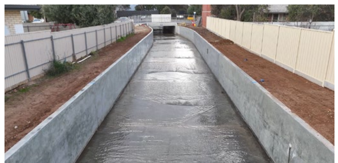
Channel construction through to completion
